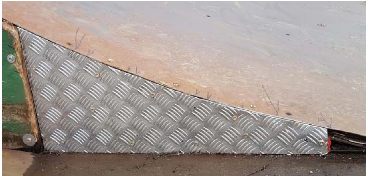
Panel replaced, will be faced in metal at a later stage
