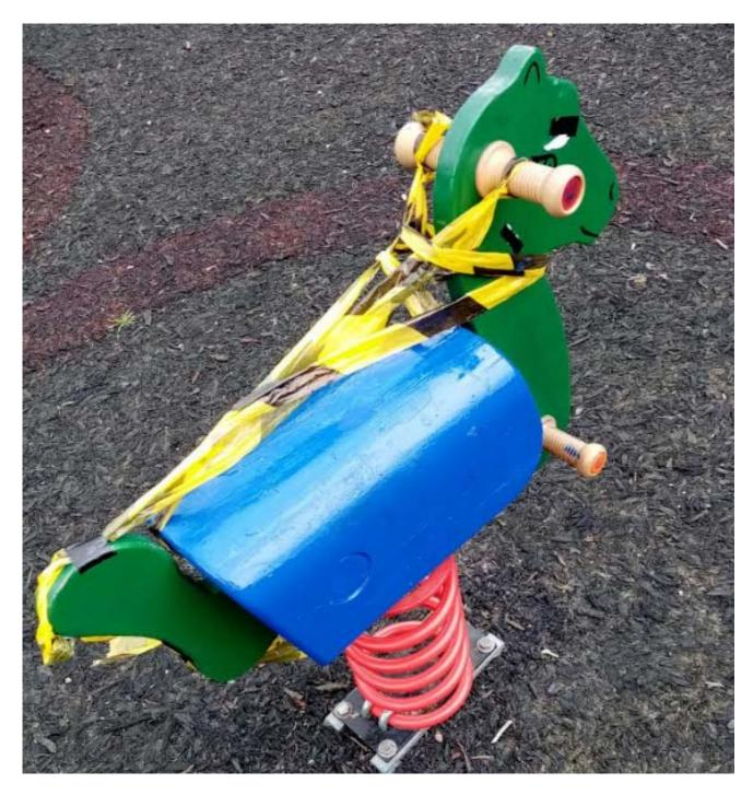
Springy horse had cracks filled with two-pack, sanded down and repainted.
