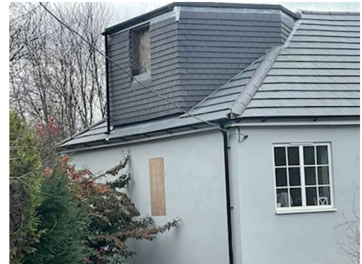
Photo of the dormer taken on 21/12.23
